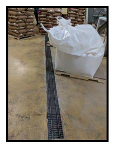
Photo 3 – View of Trench Drain in Extruder Room
