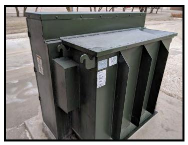
Photo 7 – View of Pad Mounted Transformer
